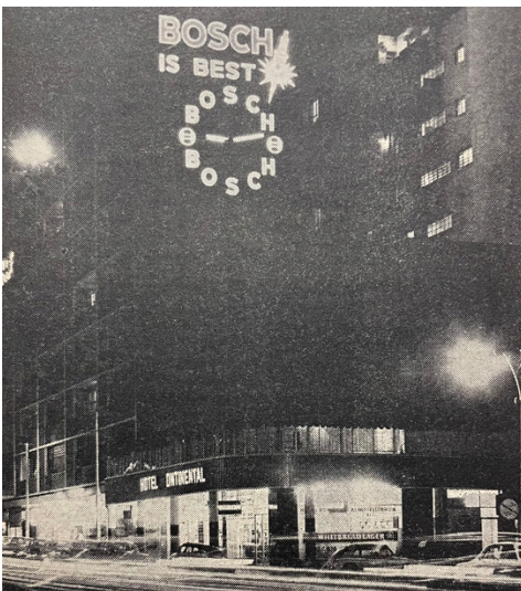
The enormous illuminated clock that Bosch had installed on a high-rise building in Johannesburg quickly became known throughout the city as the “Bosch Clock.” Photo from 1972
