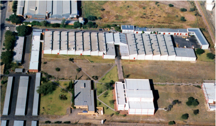
The Brits location in an aerial photograph approximately 1985: Some areas of the development site, which Bosch gradually built up to meet increasing customer demand, are still free.
