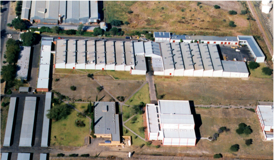
The Brits location in an aerial photograph approximately 1985: Some areas of the development site, which Bosch gradually built up to meet increasing customer demand, are still free.
