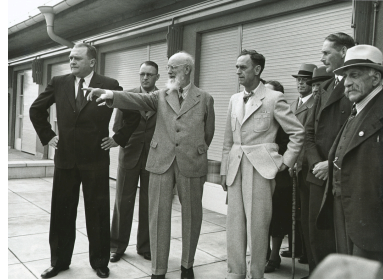
At the official opening of the Robert Bosch Hospital in 1940, Robert Bosch (third from left) proudly showed the building.
